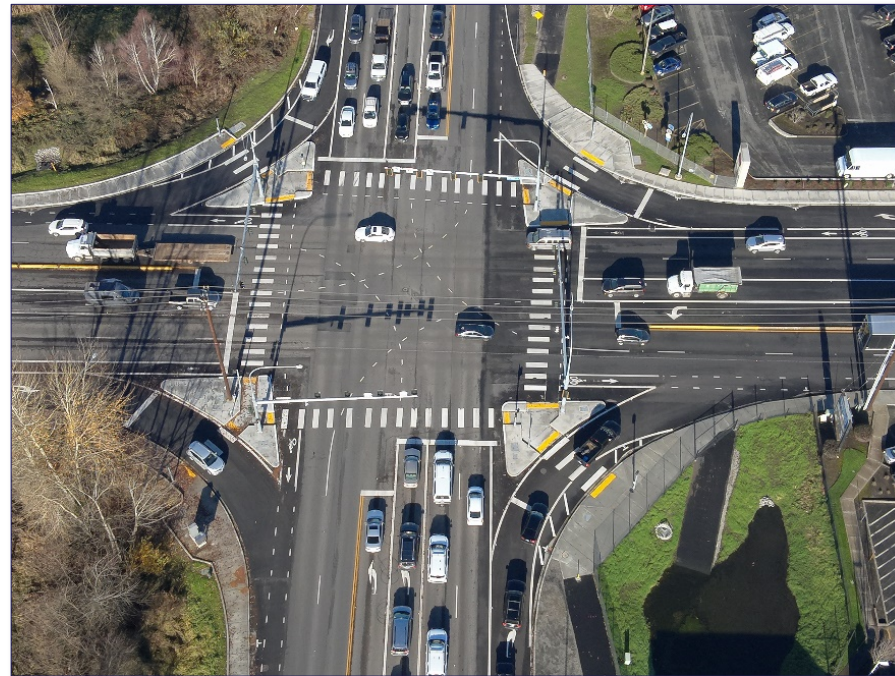
SR 502 and SR 503 Intersection
