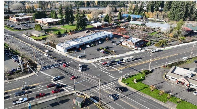
Clark County: NE 99th St. at Highway 99
