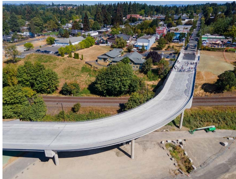
Port of Ridgefield: Pioneer Street Railroad Overpass
