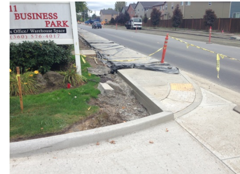
Clark County: NE 10 th Av. Construction
