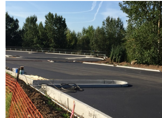
C-TRAN: Fisher's Landing Transit Center Expansion
