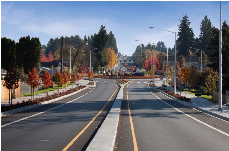
Vancouver: NE 137 th Avenue Roundabout
