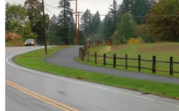
Clark County: Salmon Creek Avenue Pathway
