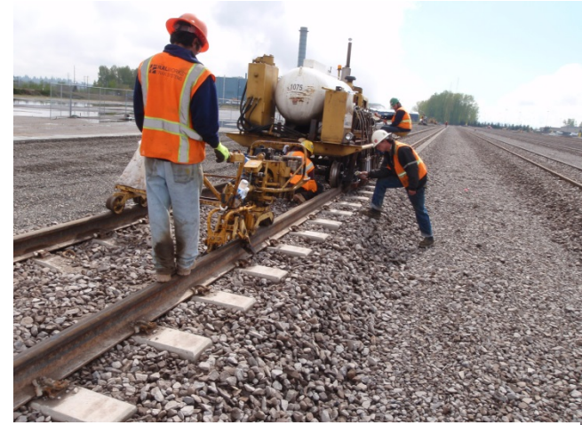
Port of Vancouver: West Vancouver Freight Access Project
