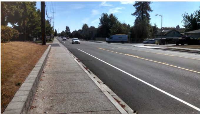
Clark County: NE 10 th Avenue, 141 st St. to 149 th St.
