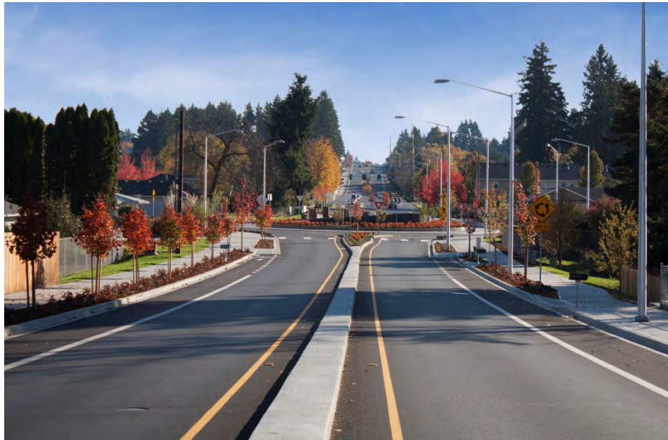
Vancouver: NE 137 th Avenue Roundabout
