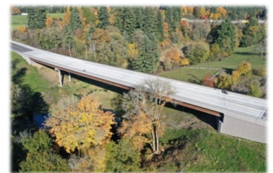
NE 10 th Ave Bridge Project
