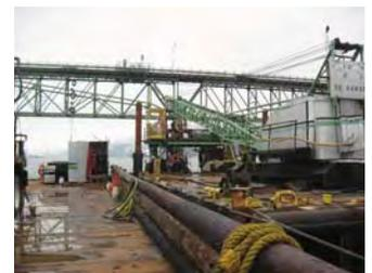
*Bridge construction will require barges and heavy cranes.*
