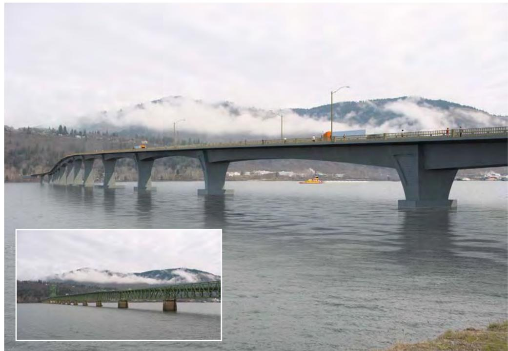
The segmental box girder option is a single box girder of varying depth constructed of concrete. This includes two 12-foot travel lanes and 8-foot shoulders, providing for a wider and safer crossing. This option has a main span of 500 feet that will yield 450 feet of horizontal navigation clearance. Segmental box girder approach spans with lengths varying from 100 feet to 400 feet will comprise the remainder of the bridge.
