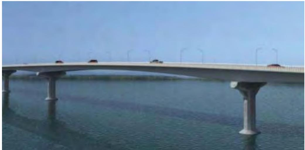
The steel plate girder option consists of multiple girders in the cross section of varying depth. Steel plate girder bridges are commonly used for typical highway crossings. For this application, longer spans were needed. This option has a main span of 500 feet that will yield 450 feet of horizontal navigation clearance. Steel plate girder approach spans with lengths varying from 75 feet to 350 feet will comprise the remainder of the bridge.
